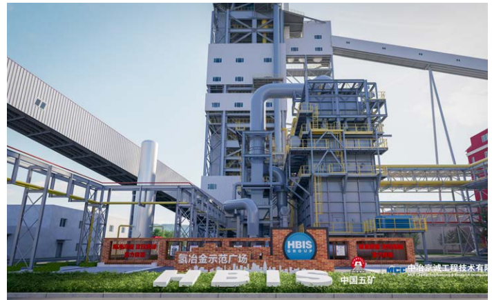
MCC CERl's digital twin cut construction time by up to three years, leading to significant cost savings.
