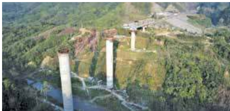
▲ The Ministry of Railways, Government of India, needed to build a 111-km rail line that includes a 141-m-tall bridge in a very active seismic area with high-speed winds and rainfall totals of 3,500 mm per year. (Image courtesy of Indian Railways).
